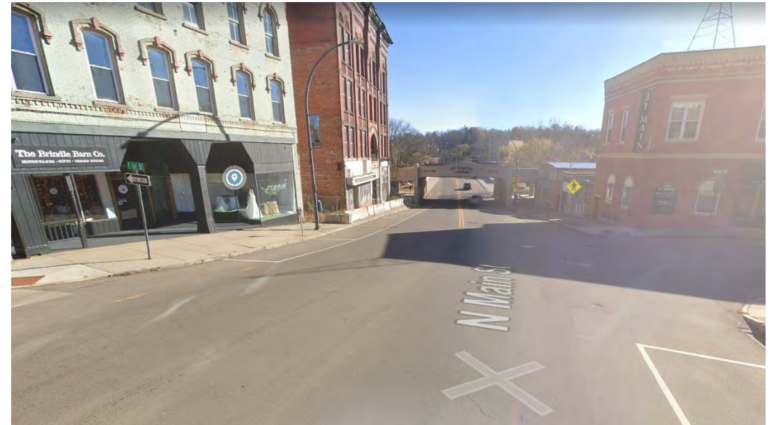
Main Street viaduct- looking south
