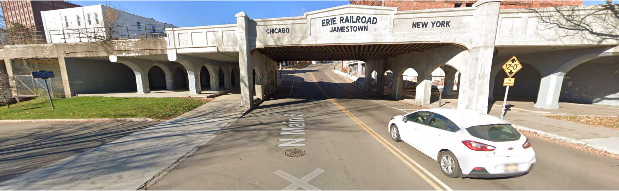
Main Street viaduct
