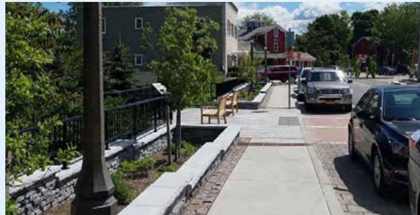
This project in Williamsville, NY, demonstrates multiple green infrastructure strategies, including permeable pavers for the parking lane and bioretention planters as part of the streetscape that capture stormwater and reduce runoff. Strategies like this also help create a more attractive environment.
