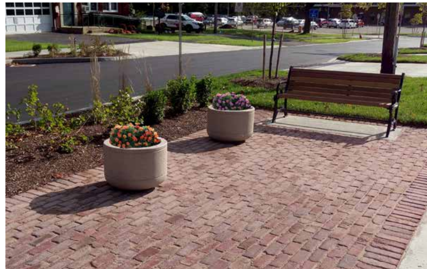
This streetscape project in Springville, NY, incorporated green infrastructure, including permeable pavers, as part of a project that relocated utilities to provide buffer space to the sidewalk and installed landscaping.
